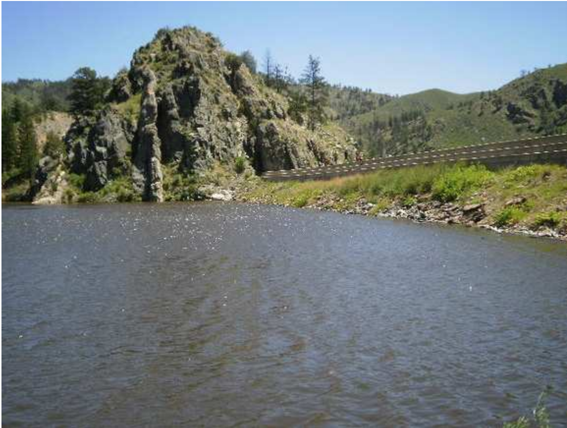
The dam is a large concrete-reinforced earth-filled design between the canyon side and this large outcropping. The spillway is on the other side. The four older kids have climbed up the nearer side of the dam, and are visible almost at the other end.
