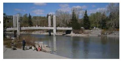
A very fancy bridge takes Centre Street over the river. Northbound traffic runs on the top of the bridge, and southbound traffic runs on the deck suspended underneath. The pedestrian path goes through an arched passage on both sides and under the lower deck.
