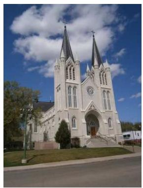
Handsome Catholic church building, Gothic Revival, but what is really interesting about it is the construction. It isn't masonry, as you might have expected. It was built in 1912 (yes, the year of Arizona statehood) by a continous concrete pour into molds, from the foundation all the way up to the towers. No joints. I'm sure it is steel reinforced (which I would think is unusual for concrete work in that era), but I can't help but wonder if they have problems with cracking and settling.
